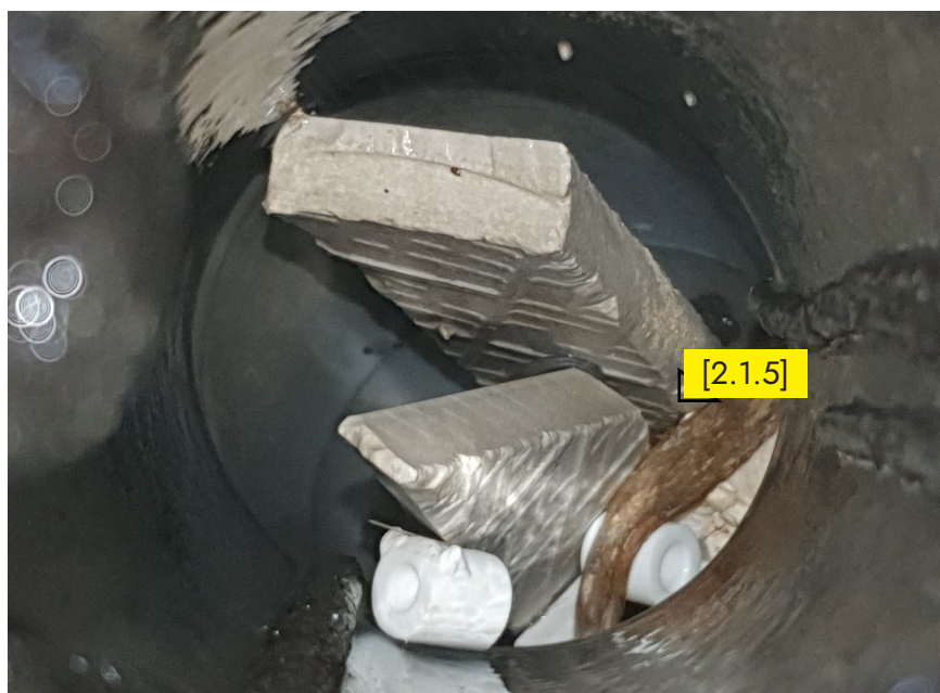
Endoscopic image of the debris in the terrace drainage pipe
